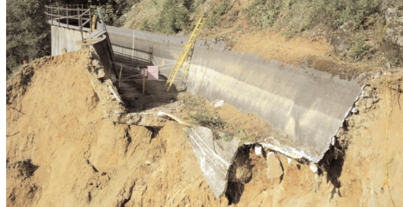
Collapsed Bear River Canal (2011)
