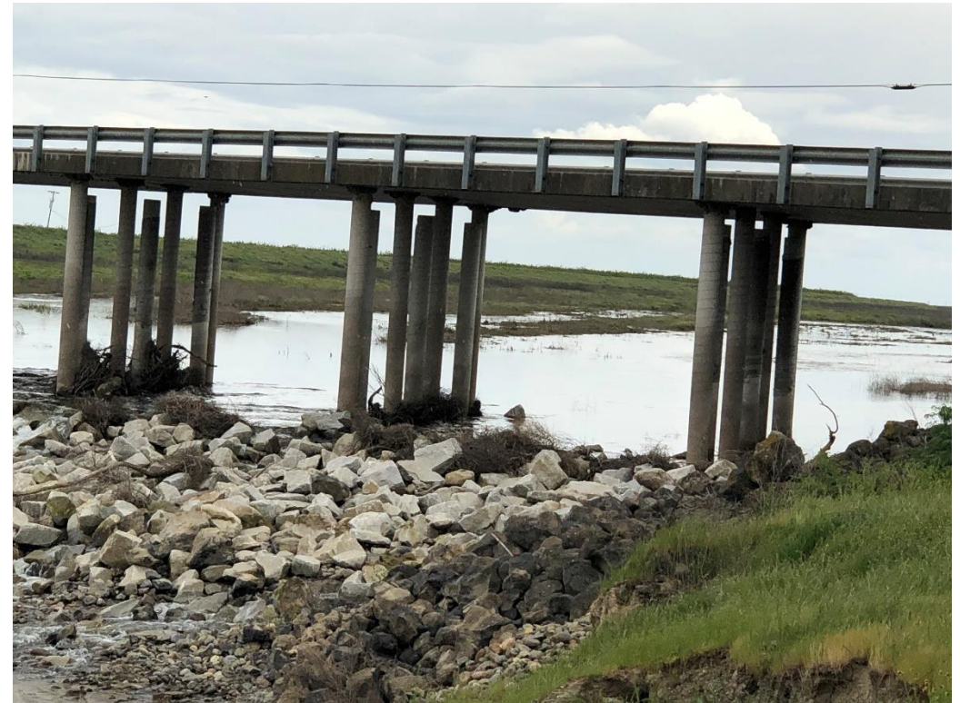
Abutments that have sank with subsidence
